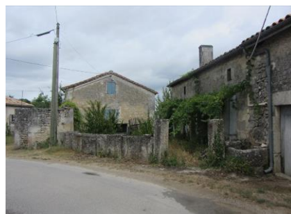
Les Balatries, Chadurie
